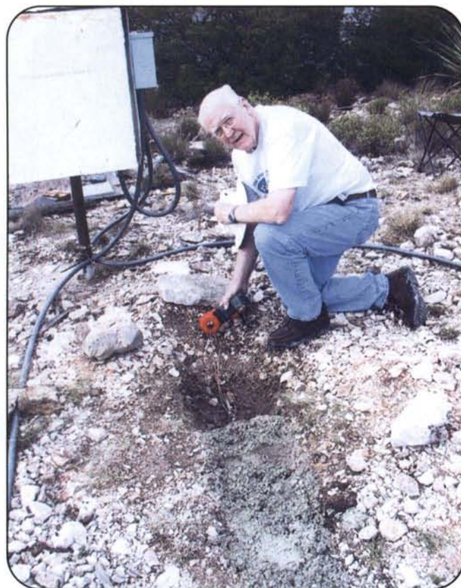
Photo 4. Joe, W5KTX, measures the resistance of the #6 ground wires attached to the copper-clad steel rod encased in the center of the 8" x 8" x 9' trench.
