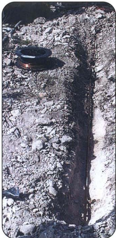
Photo 2. Shallow trench with 8' x 5/8" copper-clad ground rod propped up 4 inches.
